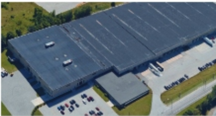
Barrie, ON (CAN) - High Performance Doors
